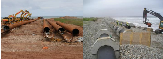
Figure 5.3 Steel (Left) and HDPE (Right) Conduits
